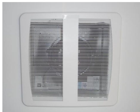
Typical Bathroom Fan
