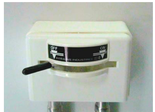
Water Shut-Off Valve
