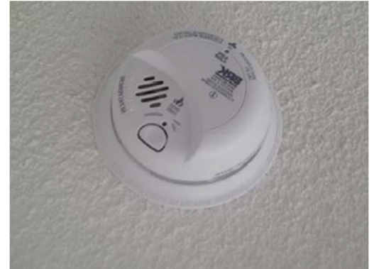
Smoke and Carbon Monoxide Detector
