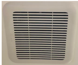
Typical Bathroom Fan
